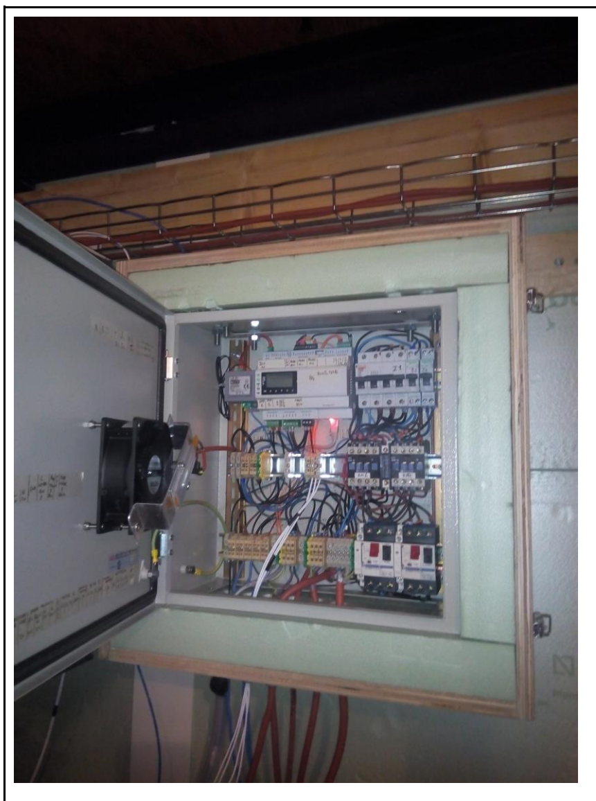
Figure 1 - Box5, mounted on the telescope building
