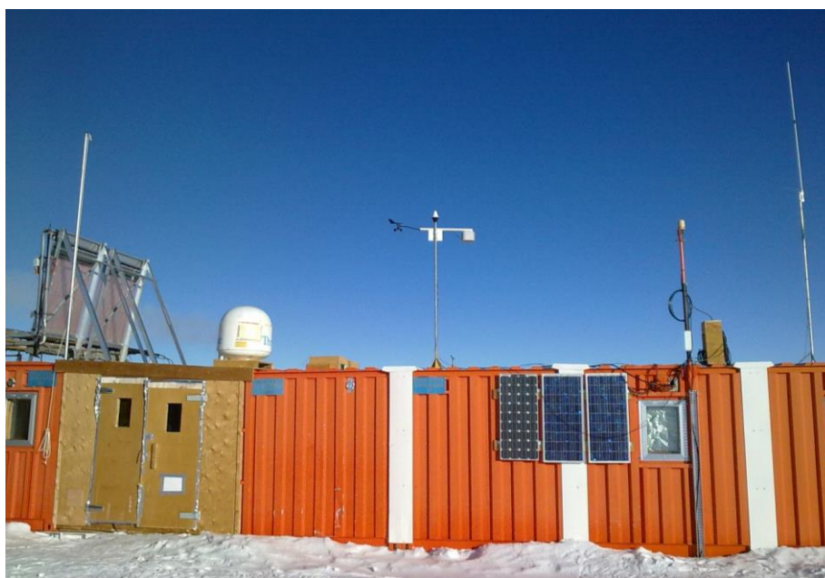
Davies Weather Station, placed on the roof of Summer Camp
