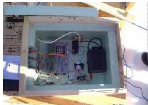
Fig. 2.2 - The new wooden box outside the shelter
