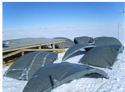
Platform and dome segments after unloading
