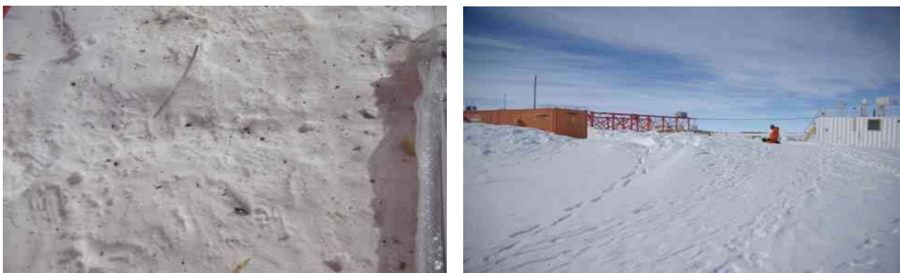
Photo 2.4 - Ground after the start of the construction of the atmospheric physics shelter, will the ground be the same during the construction of the atmospheric shelter? Position of the new structure, just in front of snowdrift. Will this site be representative of the snow of the Antarctic plateau?
